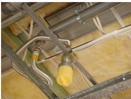
Two examples of over length flexible droppers, with excessive number of bends, or bends not meeting minimum bend radius requirements.
